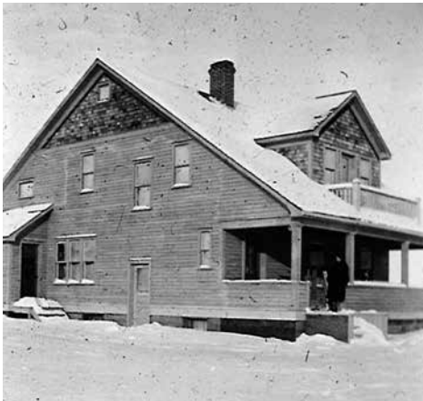
The newly constructed and yet unpainted residence of Bob & Elsie. 1932.
