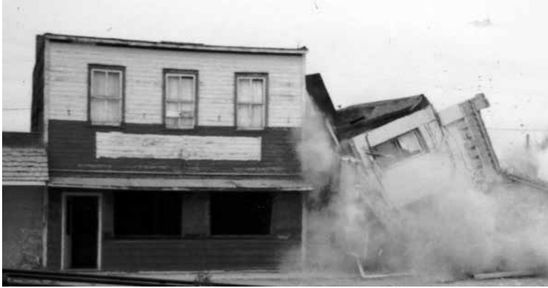
A building in Wawota, Saskatchewan, being demolished by “Boom-Boom” Geoff Hewson. 1970s.
