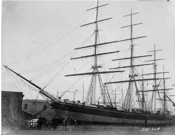
Frank Hewson's first voyage to San Francisco was on Patterdale , shown here tied up along the San Francisco waterfront. This image is from about 1880 and may be an actual image from the time he was there. North Point Warehouse, on SW corner of Sansome and Lombard, in background. Courtesy OpenSFHistory/wnp71.2322. Reprinted with permission.
